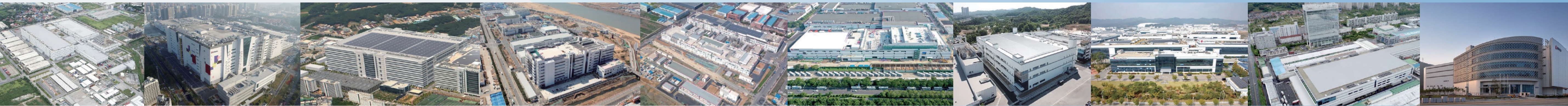
LG Display Vietnam Period: 2016.03-Present LG Display Guangzhou Period: 2015.06-Present LG Display Paju Period: 2015.10-Present LG Display Gumi Period: 2008.06-Present LG Energy Solution, Automobile battery factory in Pinkiang, Nanjing, China Period: 2018.09-2021.05 LG Energy Solution, Small battery factory in Xijiang, Nanjing, China Period: 2020.09-2022.04 LG Energy Solution Test & Research Bldg. at Ochang Factory 2 Period: 2021.06-2022.05 LG Energy Solution Ochang Factory 1 Period: 2010.07-2017.07 LG Electronics Changwon Factory 1, smart factory Period: 2018.02-2021.01 LGCNS Busan Mieum District Data Center Period: 2012.03.31-2013.01.31
